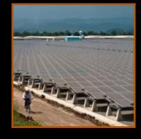
In the middle of hot and humid central Thailand, sitting on the area of more than 2 square kms, 640,000 thin-film solar panels are installed. Our SPMS supervisory system has been chosen by the global leading photovoltaic company to supervise this extra large number of panels, organized into strings, branches, sectors and connected to PV inverters and finally to the grid. Additionally, powerful O&M tools have also been provided to effectively handle such an extensive power plant.
